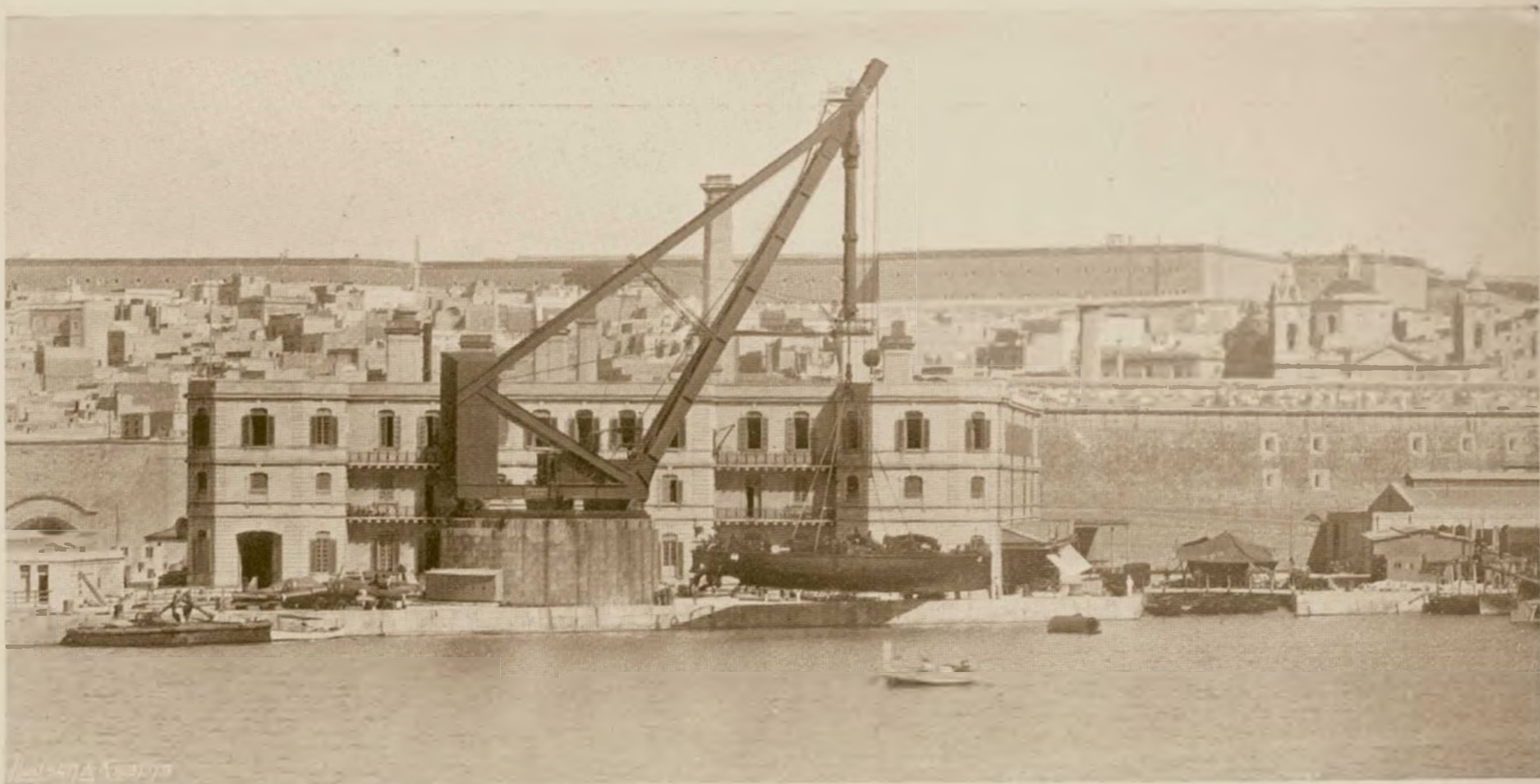
HYDRAULIC 160-TON CRANE IN FRENCH CREEK, AND VAIDALA BARRACKS.
