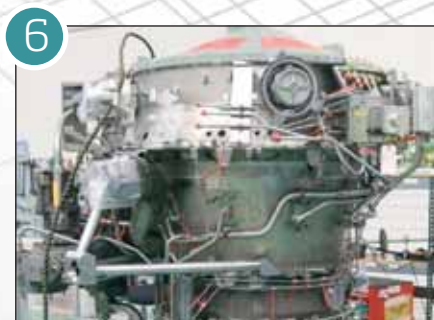
Gas turbine change unit x 2
